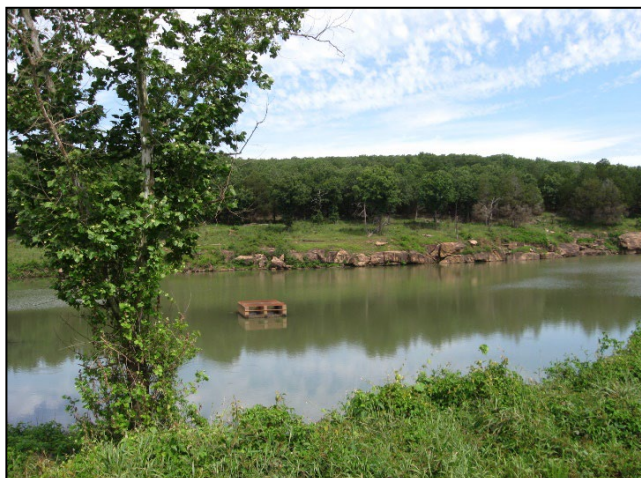
Figure No. 1 – FWRS No. 36 Existing Principal Spillway Inlet
